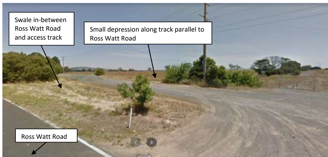
Figure 7 Depression parallel to Ross Watt Road (looking south)
